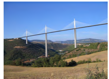
Figure H.7. Millau Viaduct in France, the highest bridge in the world. Steel and concrete, 2.5 km long and 353 m high.
