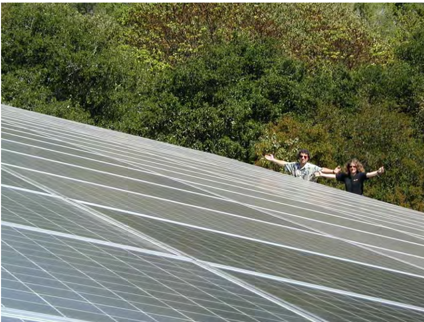
Figure 6.6. Two solar warriors enjoying their photovoltaic system, which powers their electric cars and home. The array of 120 panels ( 300\text{ W} each, 2.2\text{ m}^2 each) has an area of 268\text{ m}^2 , a peak output (allowing for losses in DC-to-AC conversion) of 30.5 kW, and an average output – in California, near Santa Cruz – of 5 kW ( 19\text{ W/m}^2 ). Photo kindly provided by Kenneth Adelman.
