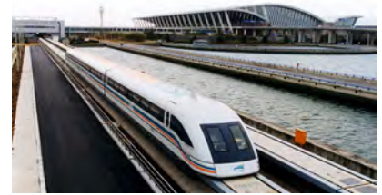
Figure 20.33. A maglev train at Pudong International Airport, Shanghai.
