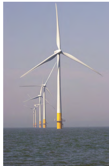
Figure 10.1. Kentish Flats – a shallow offshore wind farm. Each rotor has a diameter of 90 m centred on a hub height of 70 m. Each “3 MW” turbine weighs 500 tons, half of which is its foundation.
