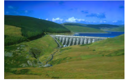
Figure 8.1. Nant-y-Moch dam, part of a 55 MW hydroelectric scheme in Wales. Photo by Dave Newbould, www.origins-photography.co.uk .
