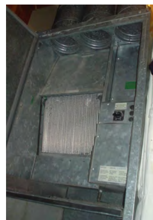
Figure E.11. The Heatkeeper's heat-exchanger.
