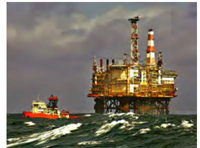
Figure 10.4. The Magnus platform in the northern UK sector of the North Sea contains 71 000 tons of steel. In the year 2000 this platform delivered 3.8 million tons of oil and gas – a power of 5 GW. The platform cost £1.1 billion. Photos by Terry Caverner.
