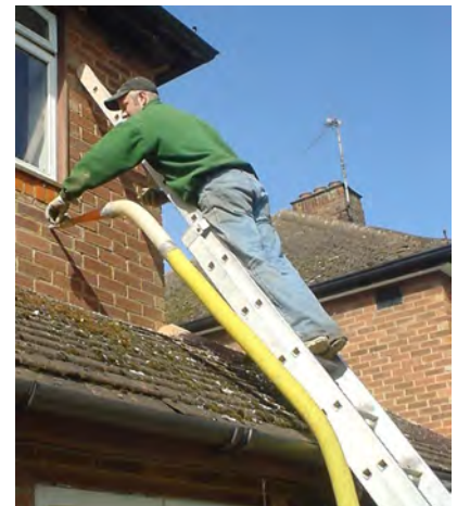
Figure 21.5. Cavity-wall insulation going in.
