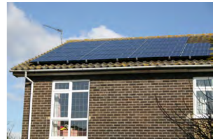
Figure 6.5. Solar photovoltaics: data from a 25\text{-m}^2 array in Cambridgeshire in 2006. The peak power delivered by this array is about 4 kW. The average, year-round, is 12 kWh per day. That's 20\text{ W} per square metre of panel.
