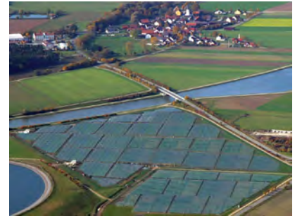
Figure 6.7. A solar photovoltaic farm: the 6.3 MW (peak) Solarpark in Mühlhausen, Bavaria. Its average power per unit land area is expected to be about 5 W/m 2 . Photo by SunPower.
