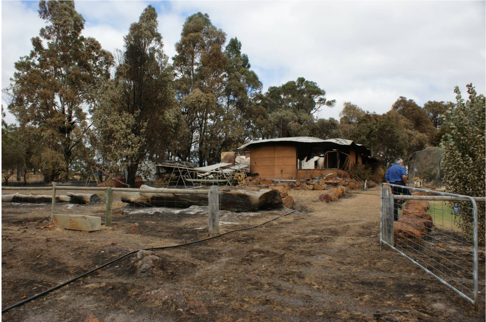
Figure 11 Burnt house in Highlands Estate. The occupant was not at home when the fire arrived. Ignition was probably due to ember attack.
