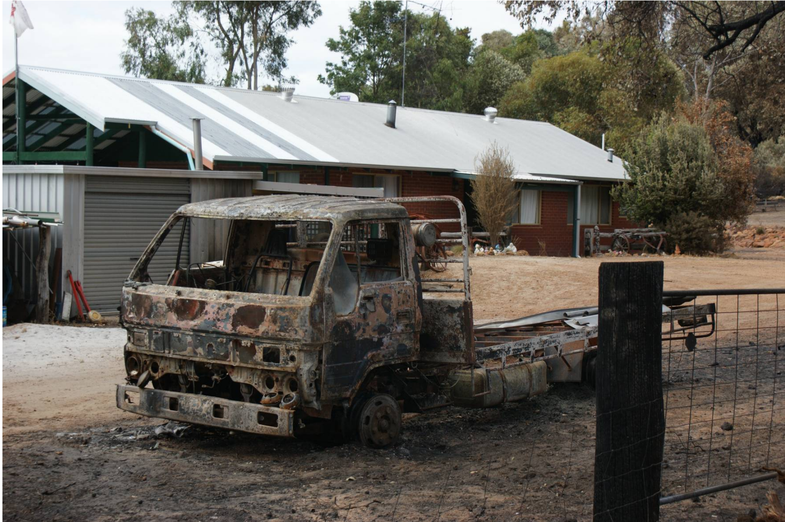
Figure 10 Burnt truck in Highlands Estate. Note minimal damage to house structure due to preparedness of occupants and defense by occupants during the fire event.
