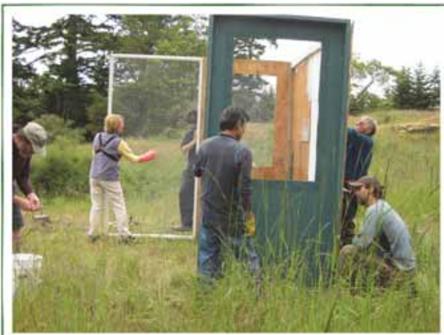
Constructing aviary © Gary Slater
