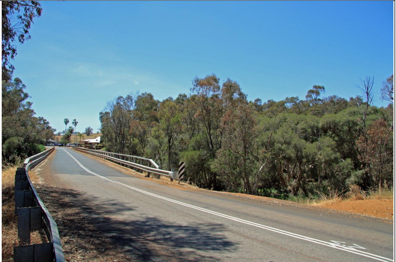
Photo point 1: Quindanning road bridge looking northeast
