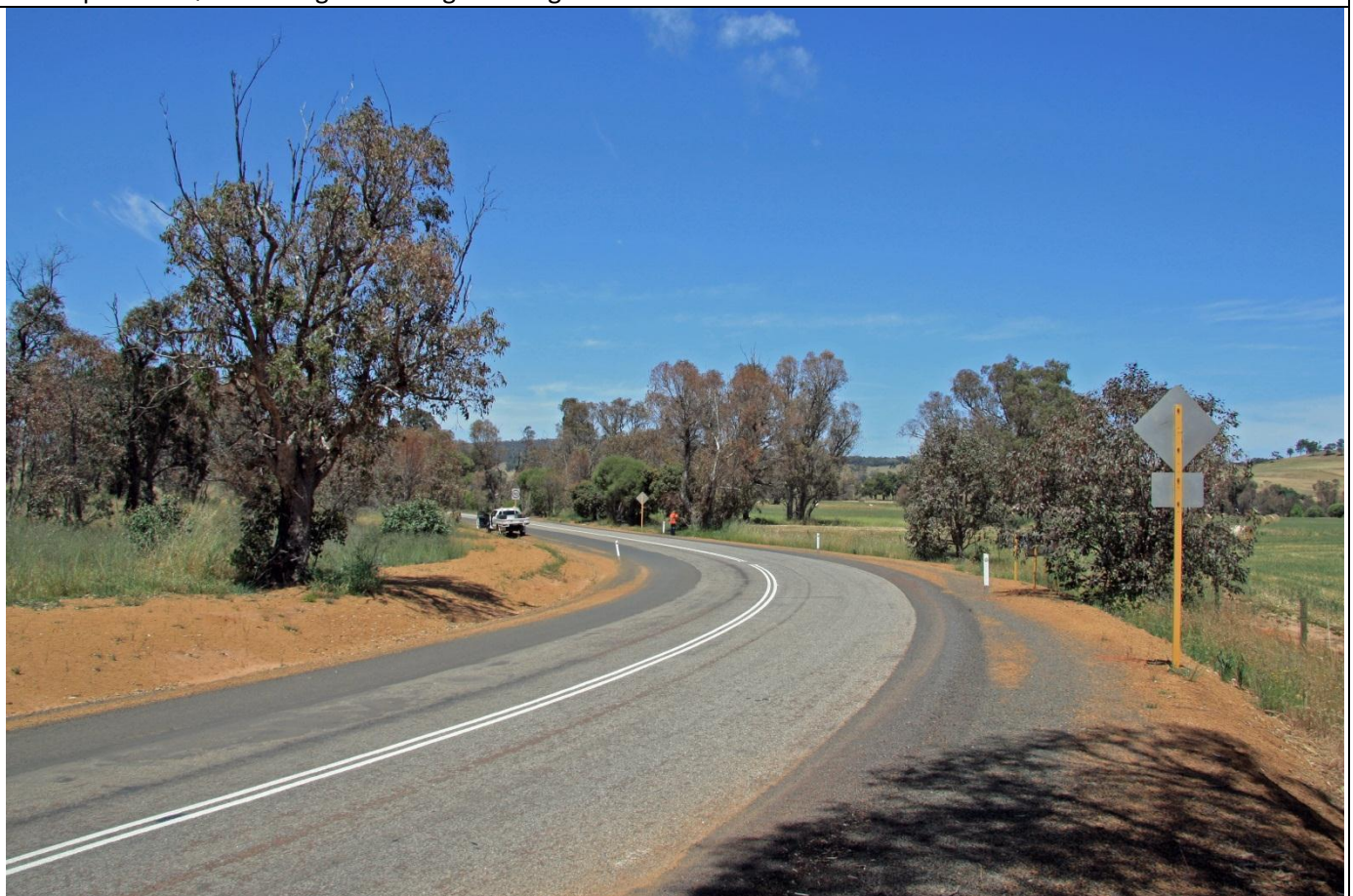
Photo point 1: Quindanning bridge looking south east
