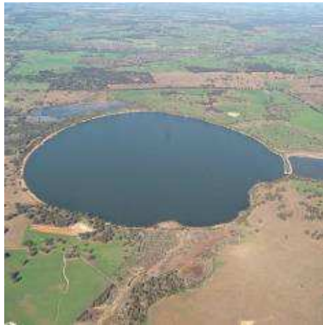
Photo 45: Towerrinning (West Arthur) water levels have been higher and salinities lower since flow diversion and other works in the early 1990s. Photo 24May2008.
