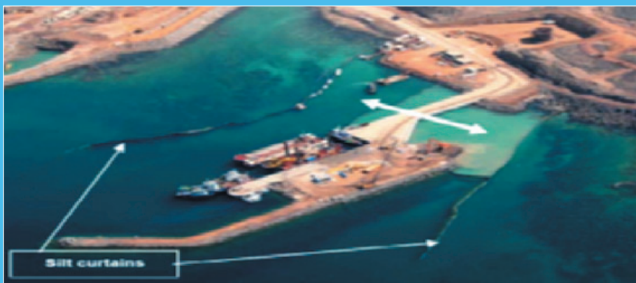
Above left: The Balhaf site showing areas impacted by the LNG jetty and intake cooling water pipelines. Above right: coral translocation in progress. Left: silt curtains deployed during LNG jetty construction.
