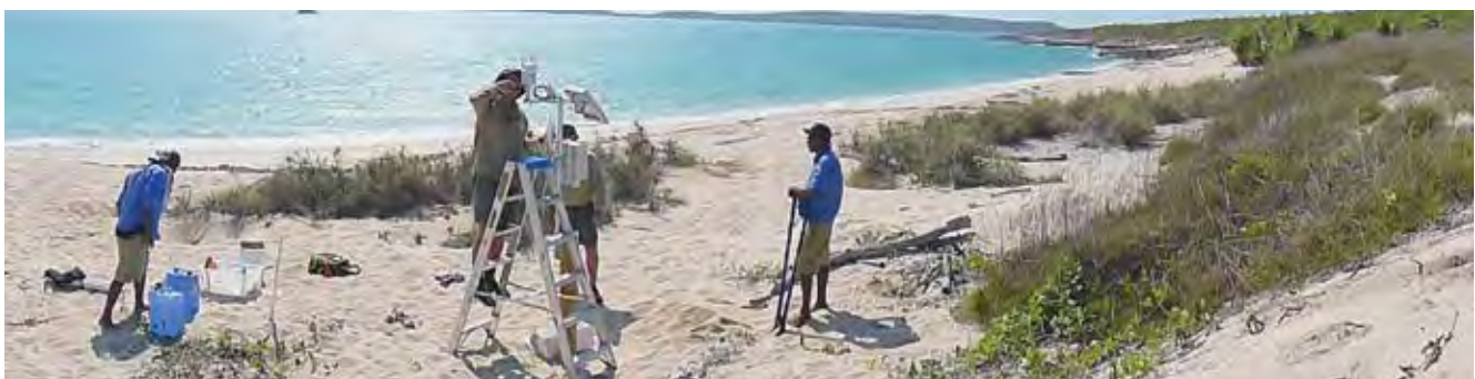
Parks and Wildlife and Dambimangari Rangers installing base and datalogger of WAMSI weather station in Dambimangari country. Photo – Michael Hourn/Parks and Wildlife
