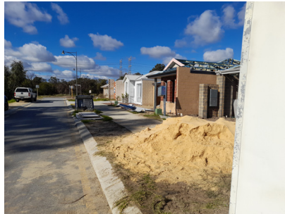
Above left: Uncovered building sand stockpile migrating onto road, Orisno Boulevard, North Coogee, City of Cockburn. (Photo credit: Lisa Brideson)
