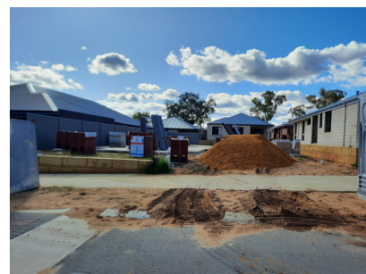
Above left: Vehicular tracking of sand west accessway Malurus St/Corocina Vista subdivision, City of Kwinana. (Photo credit: Bronwyn Scallan)
