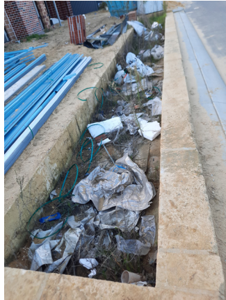
Left: Raingardens installed in new subdivision to capture sediment at Coracina Vista, Wellard subdivision, City of Kwinana, rendered significantly less effective due to littering. (Photo credits: Bronwyn Scallan)
