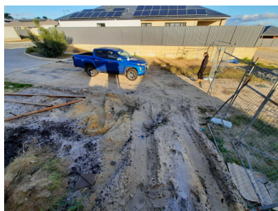
Above left: Vehicular tracking of sand west accessway Malurus St/Corocina Vista subdivision, City of Kwinana. (Photo credit: Bronwyn Scallan)
