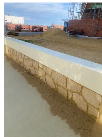
Right: Retaining wall results in sand being blown on to side over path at site on Orsino Boulevard, North Coogee, City of Cockburn, amplifying sediment loss.
