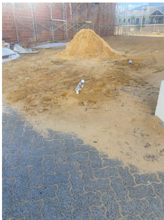
Above left: Uncovered building sand stockpile migrating onto road, Orisno Boulevard, North Coogee, City of Cockburn. (Photo credit: Lisa Brideson)
