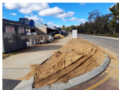
Above left: Sand tracked on road by earthmoving machinery and trucks, Lake St subdivision Rockingham, Rockingham LGA. (Photo credit: Bronwyn Scallan)
