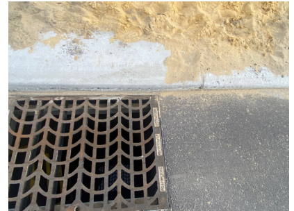
Above left: Uncovered building sand stockpile migrating onto road, Orisno Boulevard, North Coogee, City of Cockburn. (Photo credit: Lisa Brideson)
