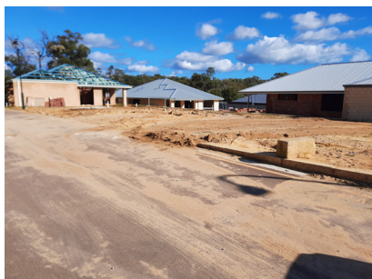
Above left: Vehicle tracking of sand onto roads from residential building site in Bolam Lane, Wellard, a new subdivision in the City of Kwinana. (Photo credit: Bronwyn Scallan)
