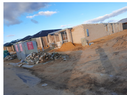
Above left: Vehicle tracking of sand onto roads from residential building site in Bolam Lane, Wellard, a new subdivision in the City of Kwinana. (Photo credit: Bronwyn Scallan)
