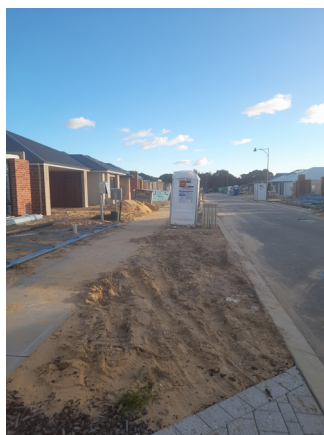
Above left: Vehicle tracking of sand onto roads from residential building site in Bolam Lane, Wellard, a new subdivision in the City of Kwinana. (Photo credit: Bronwyn Scallan)
