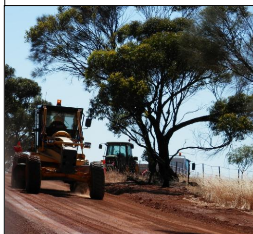
Care must be taken when clearing to ensure large trees are not damaged, that the clearing is actually necessary and that the required permits are obtained. Photos: RCC
