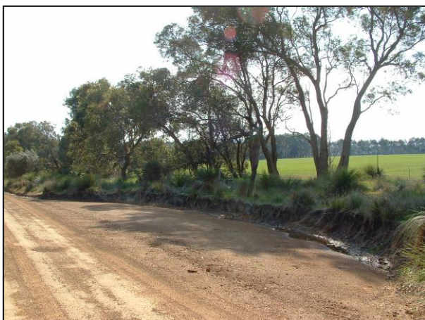
Creative solutions: A high value Flora Road in the Shire of Plantagenet. Passing lanes were established at various locations along the road to eliminate the need for widening the whole road. Photo: C. Macneall, RCC.
