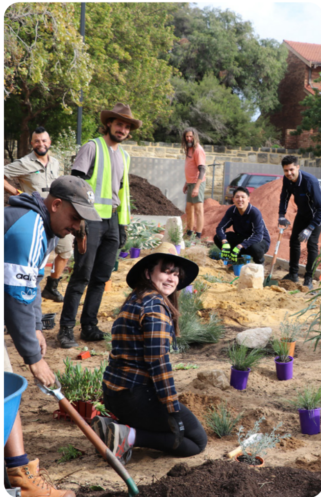
Waterwise landscaping in progress
