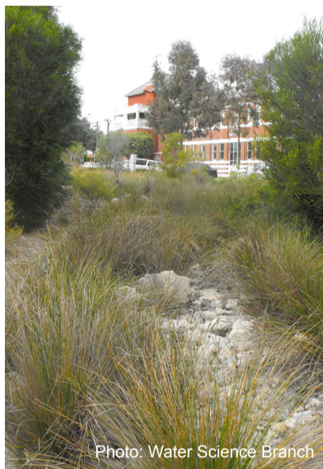
Stormwater treatment in drainline at Robertson Park, August 2010.
