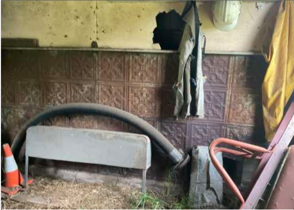
Room 1 northern dado panelling
