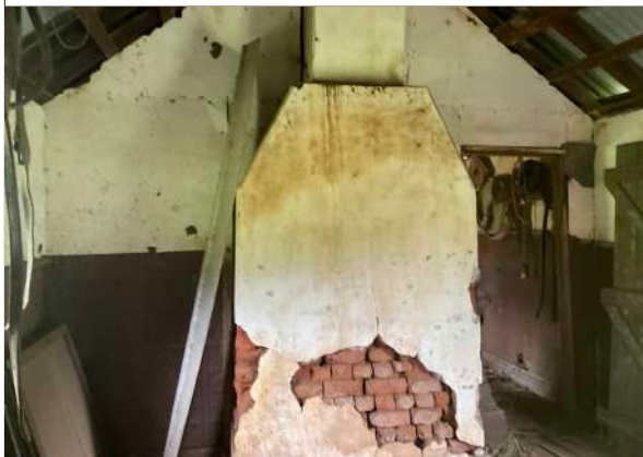
Room 2 north internal elevation
