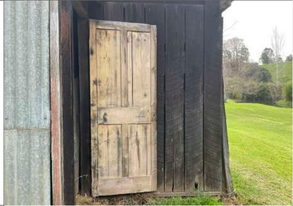
Timber door to attached external earth closet
