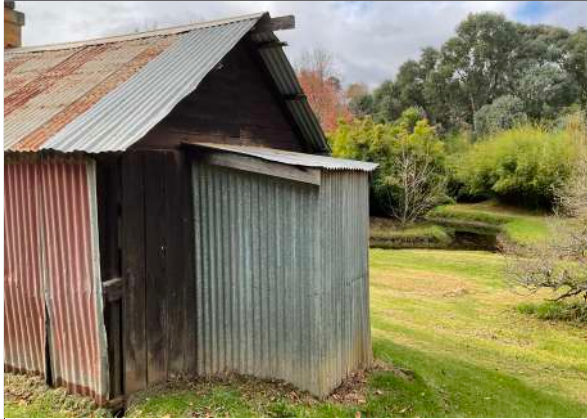
External earth closet attached to the southern elevation
