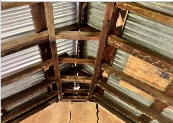
Room 1 roof structure
