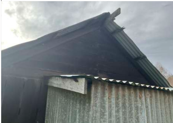
Timber boards to southern gable
