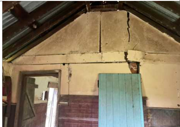
Room 1 southern wall
