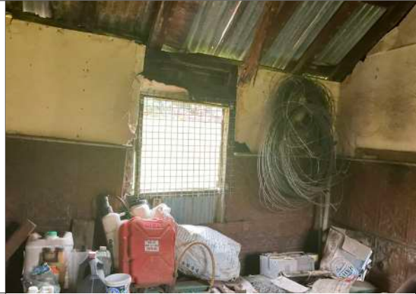
Room 1 north west corner
