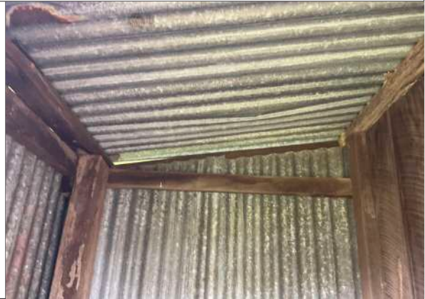
Internal structure to earth closet
