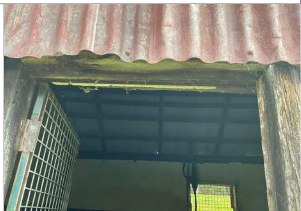
South East entry door frame
