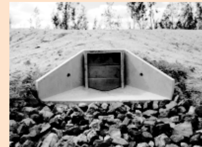
Outflow pipe on side of diversion wall
