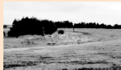
Revegetation planted along surface drain
