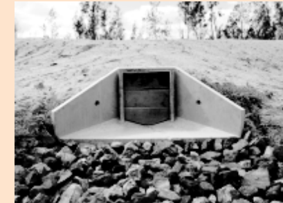
Outflow pipe on side of diversion wall
