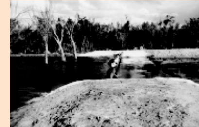
Separator gate prevents salt water flowing into the Lake
