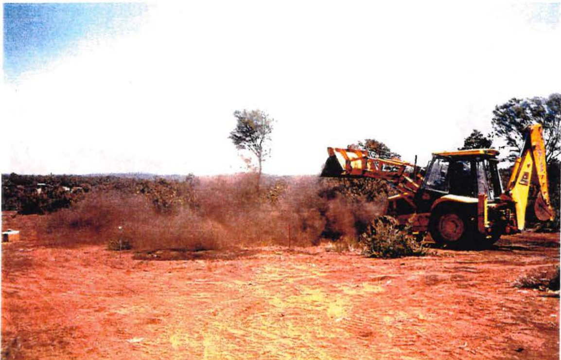
Photo 4: Trial excavation at Site C "dry".
