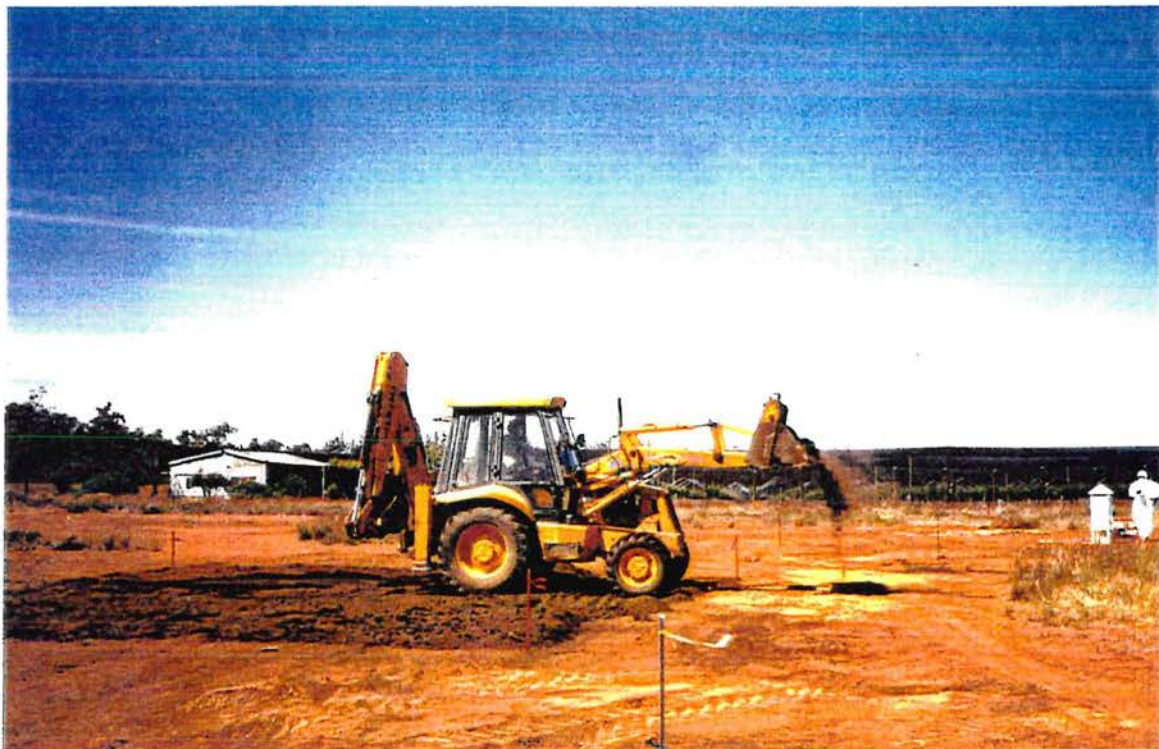
Photo 2: Trial excavation at Site A "wet".
