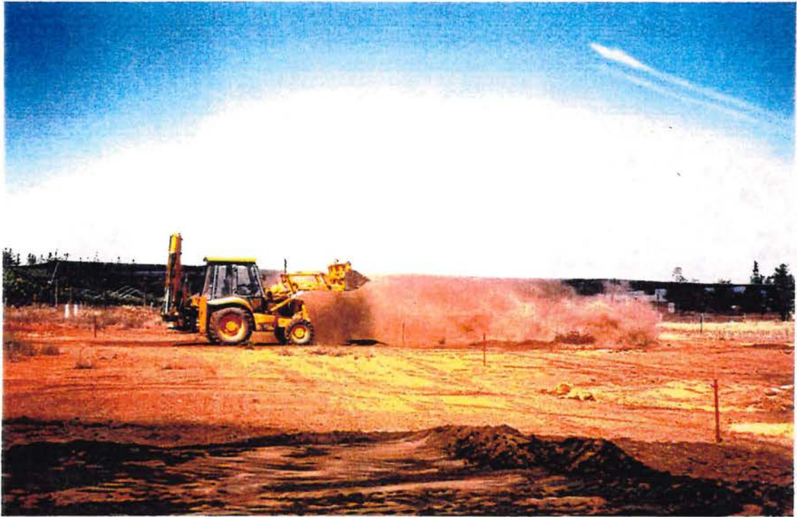
Photo 3: Trial excavation at Site A "dry".
