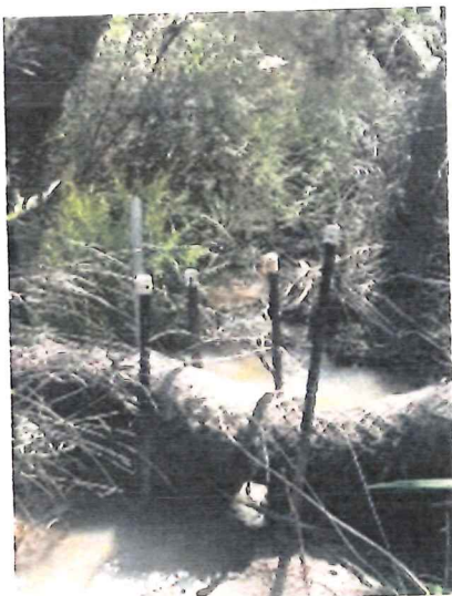
Figure 53: Coir logging in a pool downstream of Mundaring Weir Road.
