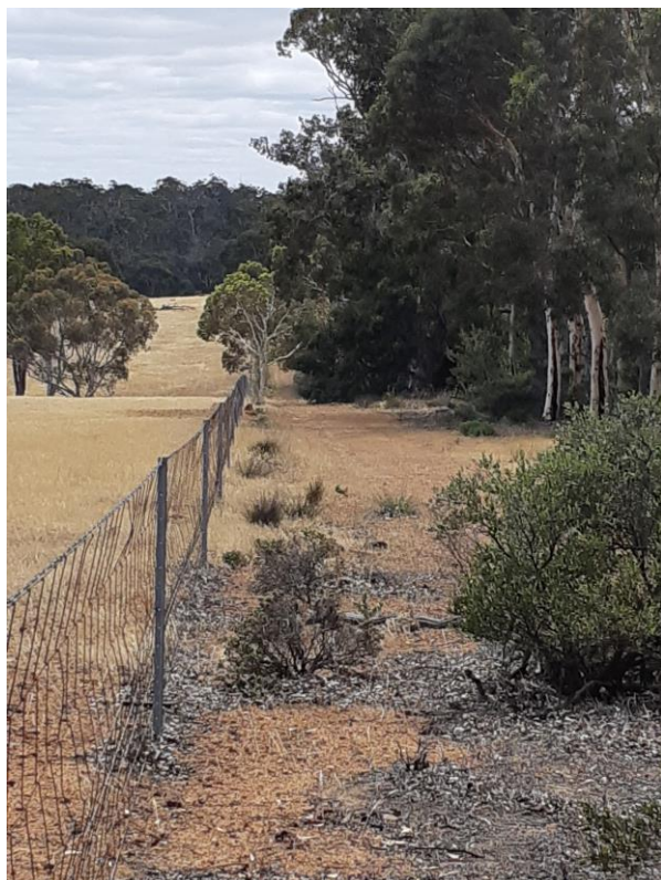
Photo 20: Fence in good condition along the southern boundary
