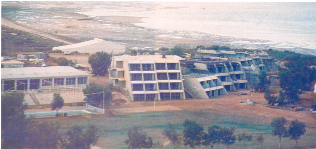
Wapet camp showing mess (L) accommodation units (R), outdoor games area and landscaping
