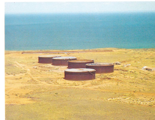
Tank farm with ballast pit behind
