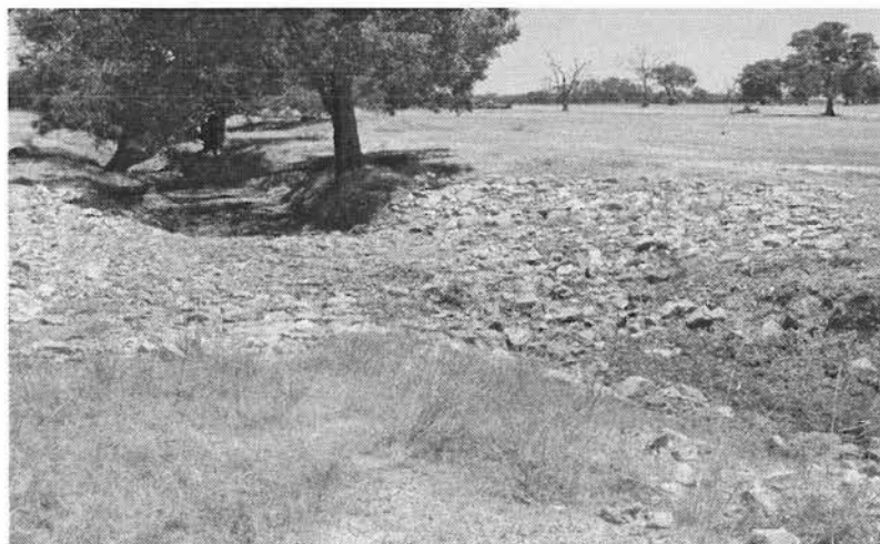
Plate 1: Placement of rocks in the drain. Photo by Cathy Lyons.
