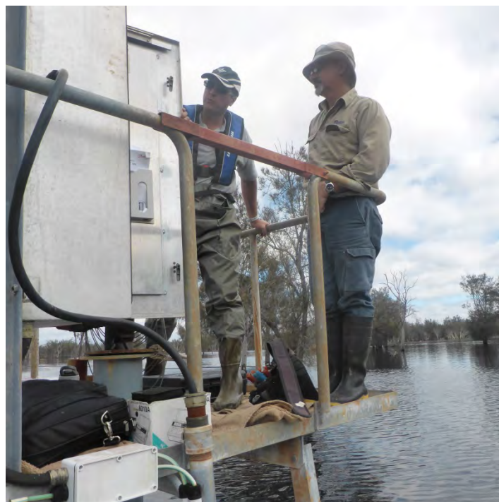
Maintenance of electric submersible pump Photo – Maria Lee/DBCA
