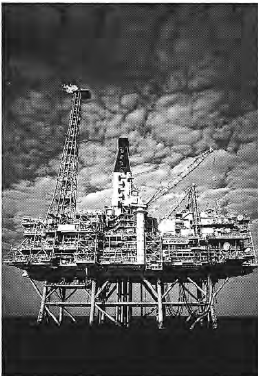
Oil and Gas production from the North West Shelf is expanding, confirming the regions position among the most economically significant land or sea regions in Australia.
