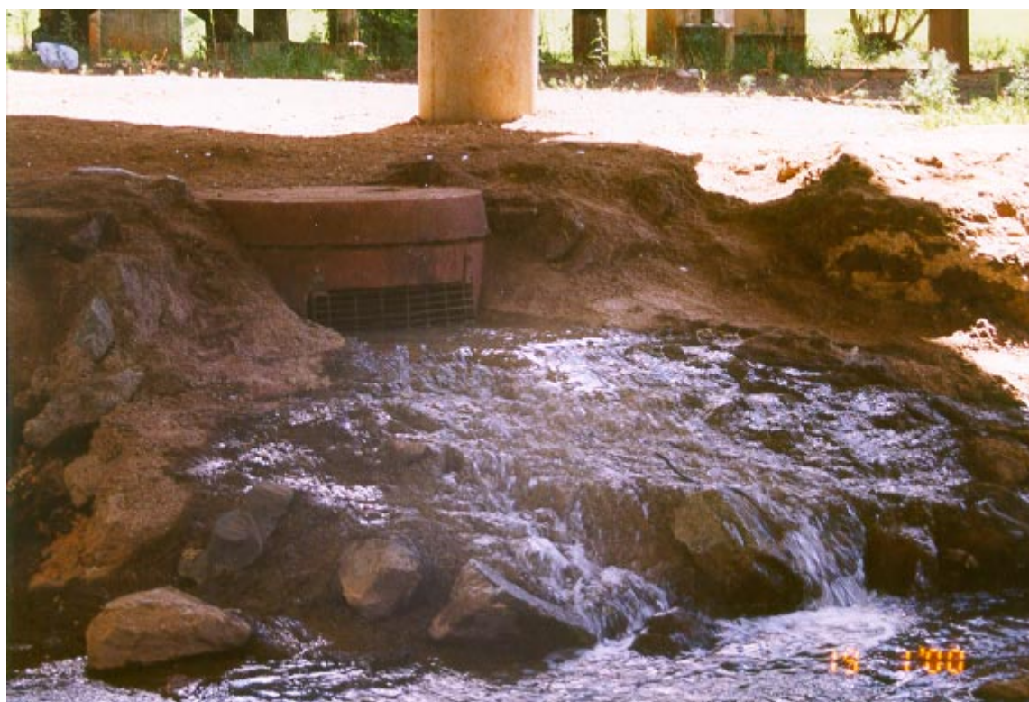
Environmental release point, Albany Highway Bridge, Gosnells
