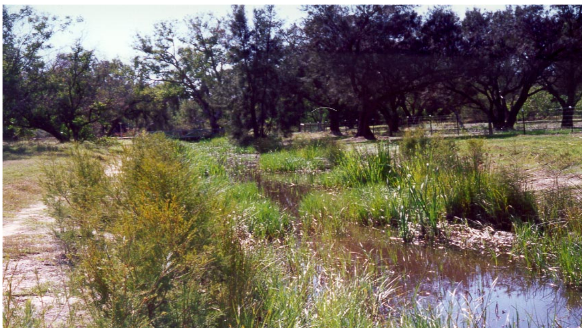
Menzies Drain, Cannington: an example of a drain being modified into a 'living stream' Photo: R Paice
