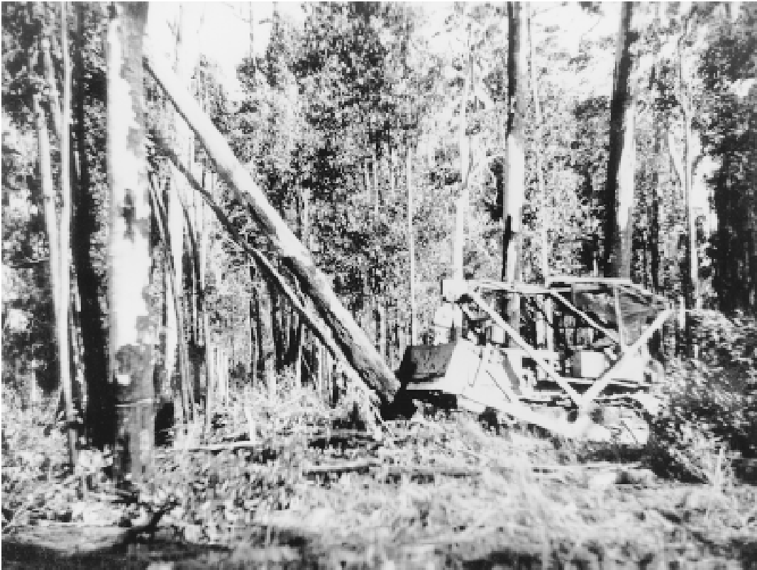
Hi-ball 'dozer clearing Jarrah in the Denmark area, 1952; Batty Library 51213P.
