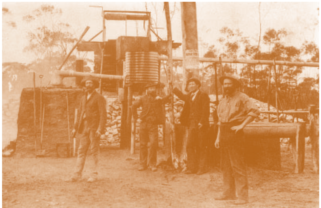
Railway condenser and operating team, c. 1895; from Le Page, 1986.
