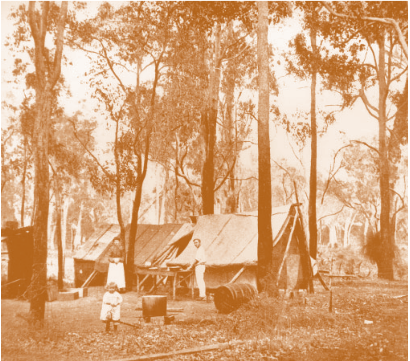
A new base for a pioneer family in the Brunswick district (pre-1920); from Brady, 1918.
