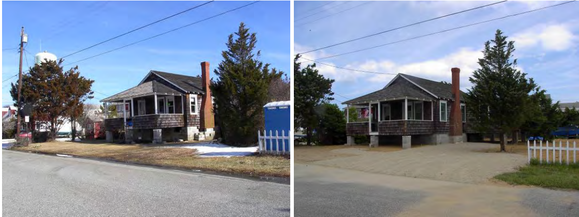
7819 Figure 12.5 Elevating land and house. (a) Initial elevation of house in Brant Beach (New Jersey). (b) 7820 Structural beams placed under house, which is lifted approximately 1.5 meters by hydraulic jack in blue 7821 truck. (c) Three course of cinder blocks added then house set down onto the blocks. (d) Soil and gravel 7822 brought in to elevate land surface. (January through June 2005) 7823
