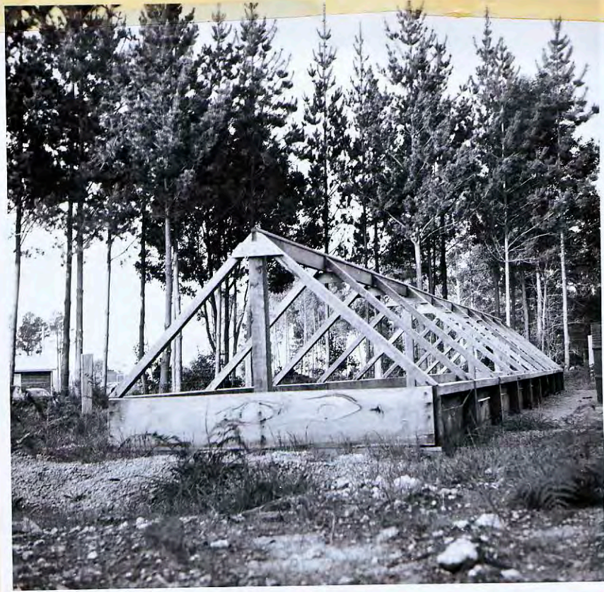
Standing out frame at Mij Research Nursery with loam floor. (Frame treated with sodium pentachlorophenol drench applied with floor mop).
