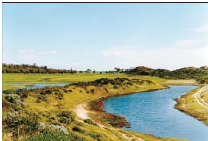
Figure 14. A drainage channel near the southern sector of Cable Sands, which could provide a good option for discharging used water.
