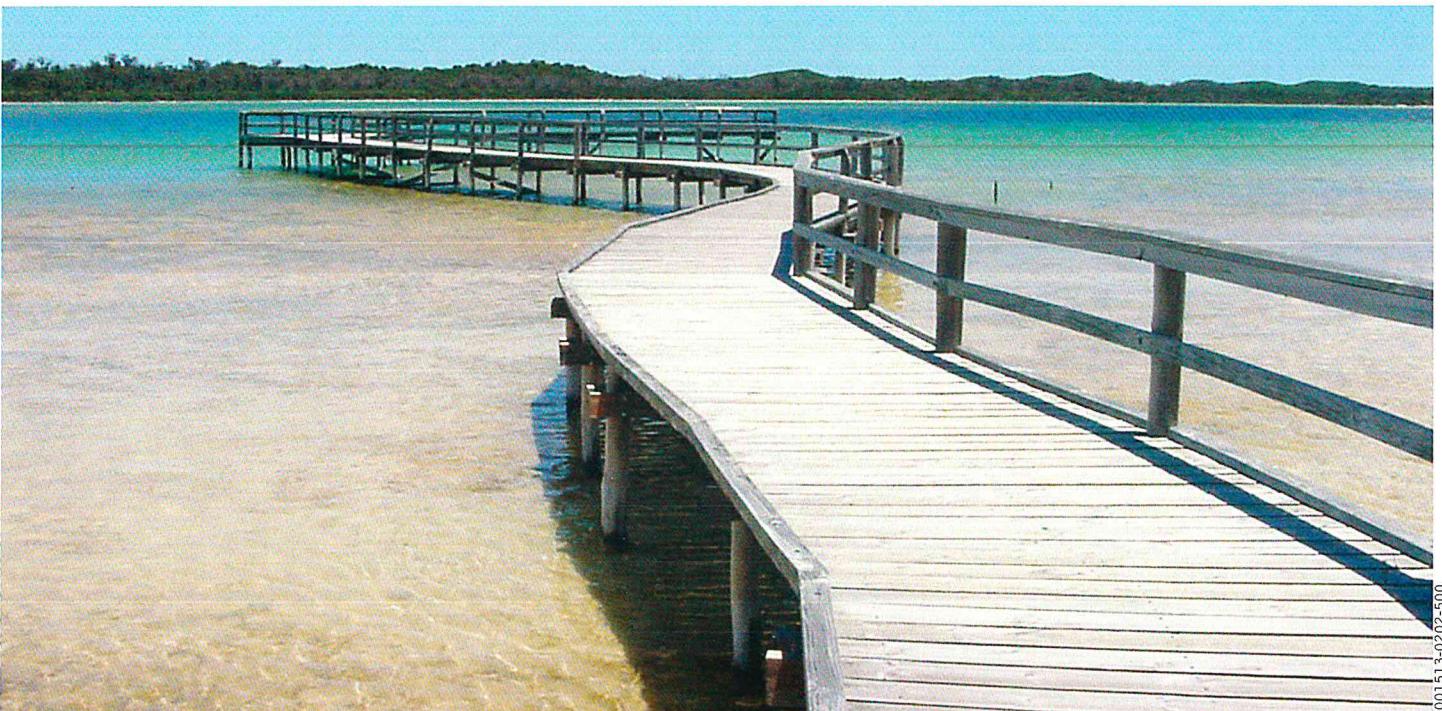
The boardwalk constructed at Lake Clifton helps prevent crushing of the thrombolites. Photo – Stephen Dutton
