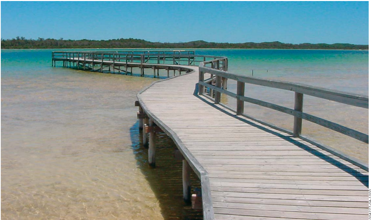
The boardwalk constructed at Lake Clifton helps prevent crushing of the thrombolites. Photo – Stephen Dutton
