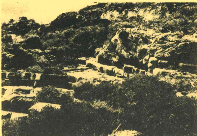
1. Conspicuously bedded aeolian limestone near Bunkers Bay. Thick, hard layers of heavily calcified limestone are interbedded with softer, poorly cemented limestone; the latter has eroded away, leaving distinct gaps between the layers.
