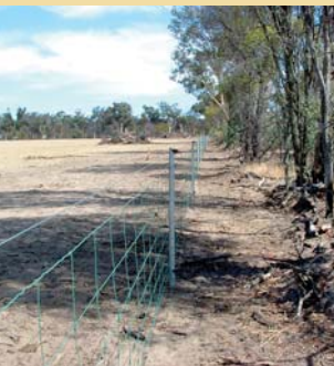
Careful clearing to minimise the impact of replacing the fence. Photo C. Wilson
