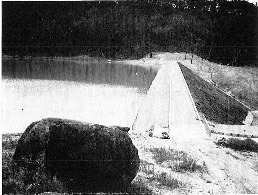
Glen Brook Dam, John Forrest National Park, W.A. (Constructed 1965)
