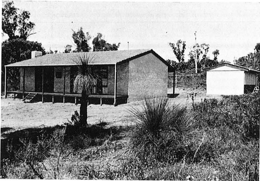
Staff House at Yanchep Park
