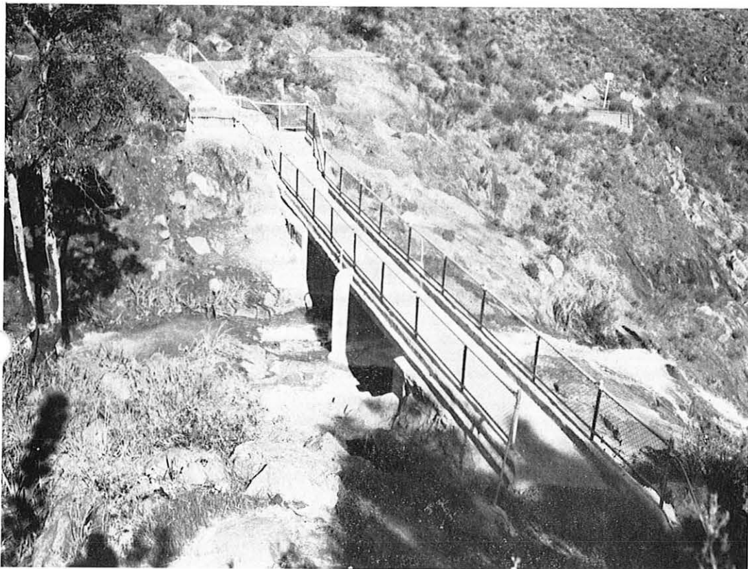
Footbridge above Lesmurdie Falls
