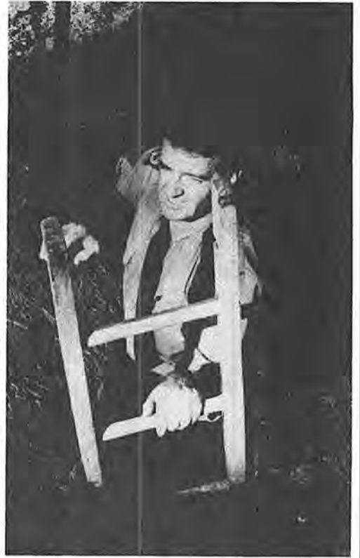
JIM MAHER squeezes through the broken hole in the tunnel roof to investigate conditions below.
