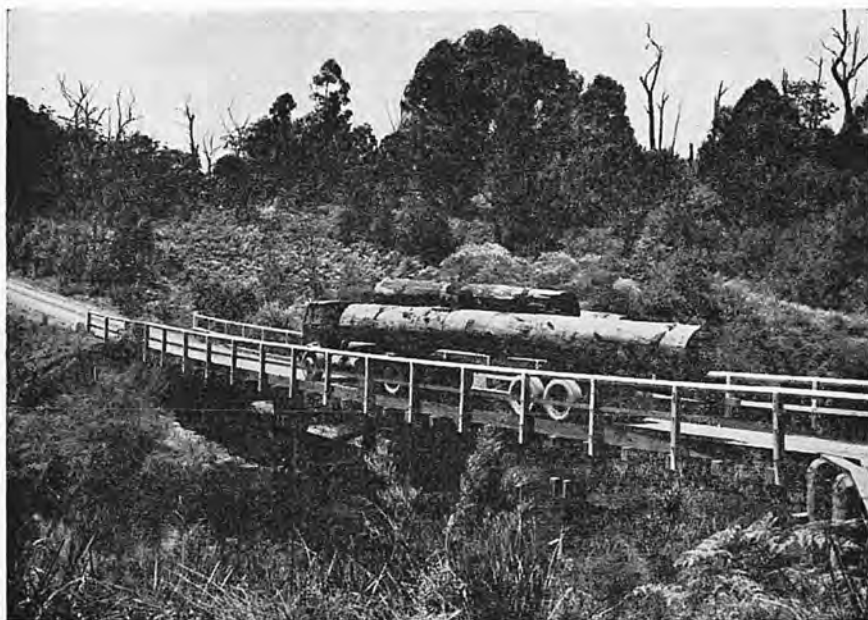
Plate 50. Motor lorries have largely replaced steam locomotives for hauling logs from the bush landing to the mill.
