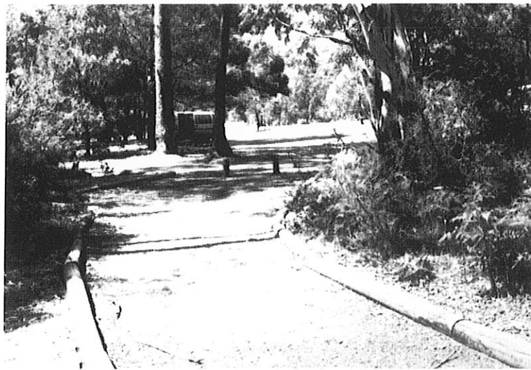
Figure 5 Carpark and main entry path to koala enclosure - Tidbinbilla Nature Reserve. Very high use area - large bitumen carparks, wide well-defined free draining access path.
