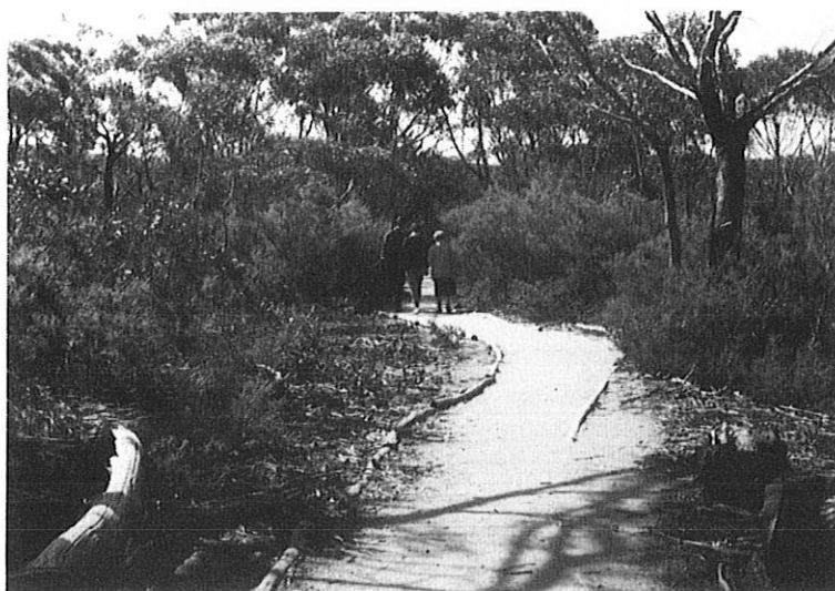
Figure 1 Walk-trail to view Kanangra-Walls. Good hard surface of decomposed granite, drains very well; wheelchair access; good width. Some rehabilitation work can be seen to the left of the path.
