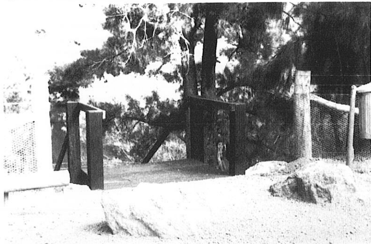
Figure 9 Stairway to river and barrier fencing (note barbed wire). Erosion from multiple access points was a problem here, but the fence and stairs have solved this. The two large rocks prevent cars from parking too close and blocking access. The stairs are made of jarrah.
