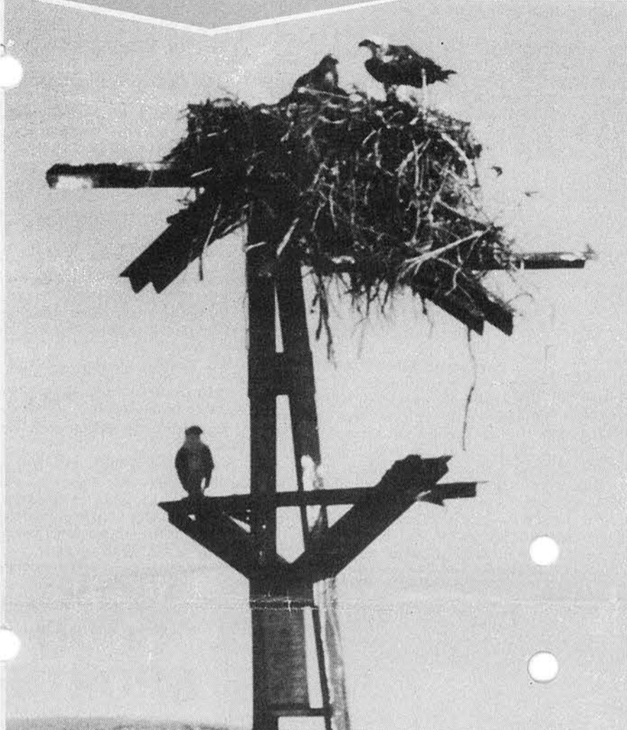
OSPREYS nesting on the old lead light tower at "Point Samson". The structure was originally used to help guide ships into the Pt. Samson jetty. Story, more pictures page 3.
