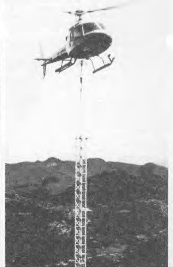
A helicopter is used to site an aerial in Tasmania.
