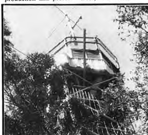
New steel reinforcements at the top of the Gloucester Tree.
