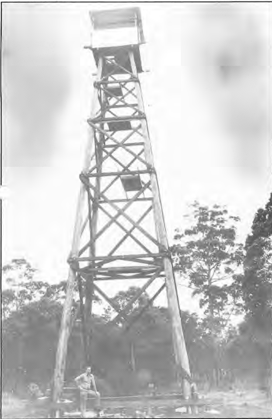
Sixty feet (from a 1936 blueprint) of forest protection. A traditional fire tower build for the Timber Park at Manjimup. (Photo courtesy Warren Blackwood Times)
