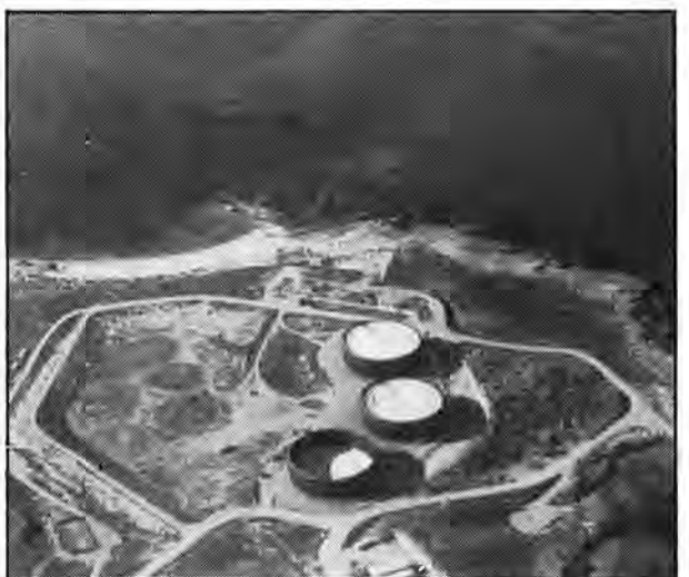
BOND'S tank farm with three 250,000 litre barrel tanks and the large emergency bund. To the top of the photo can be seen the pipeline heading out to the rig.
