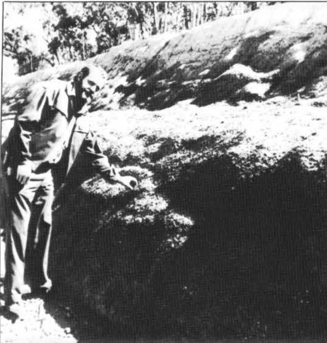
Ross McGill shows how the seeded clover has started to stabilise the carpark bank.
