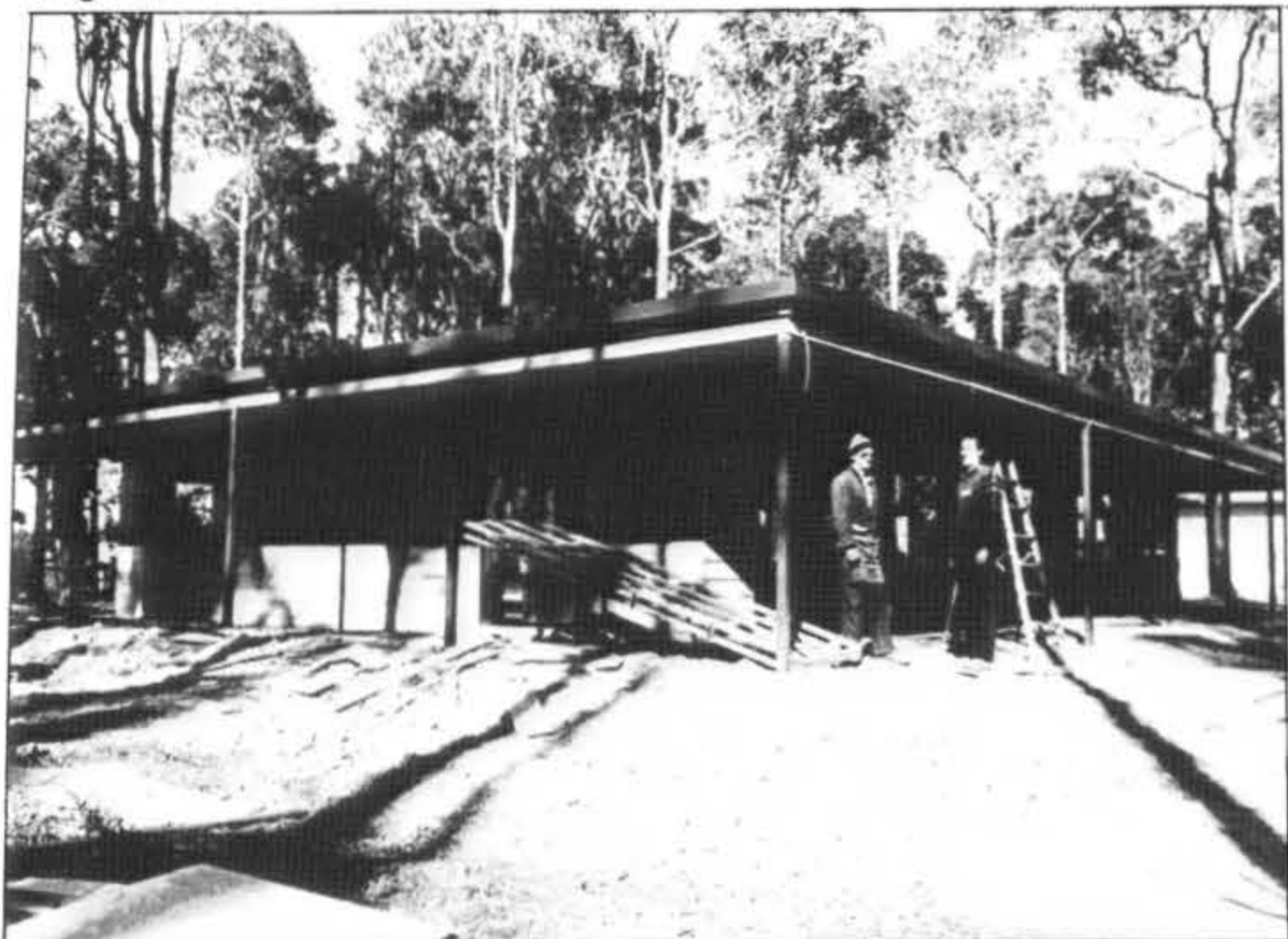
Administration building, Manjimup Nursery. Private contractor, Doug Hill (left) and Senior District Forest Officer, Peter Beatty. (Photo: Steve Murnane)
