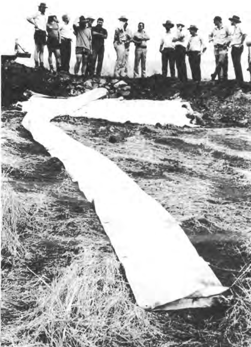
Workshop participants involved in roadwork construction
