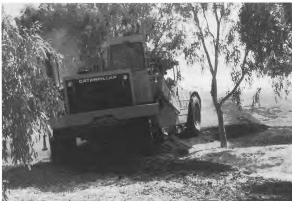
A bulldozer lays the groundwork for an interceptor bank.
