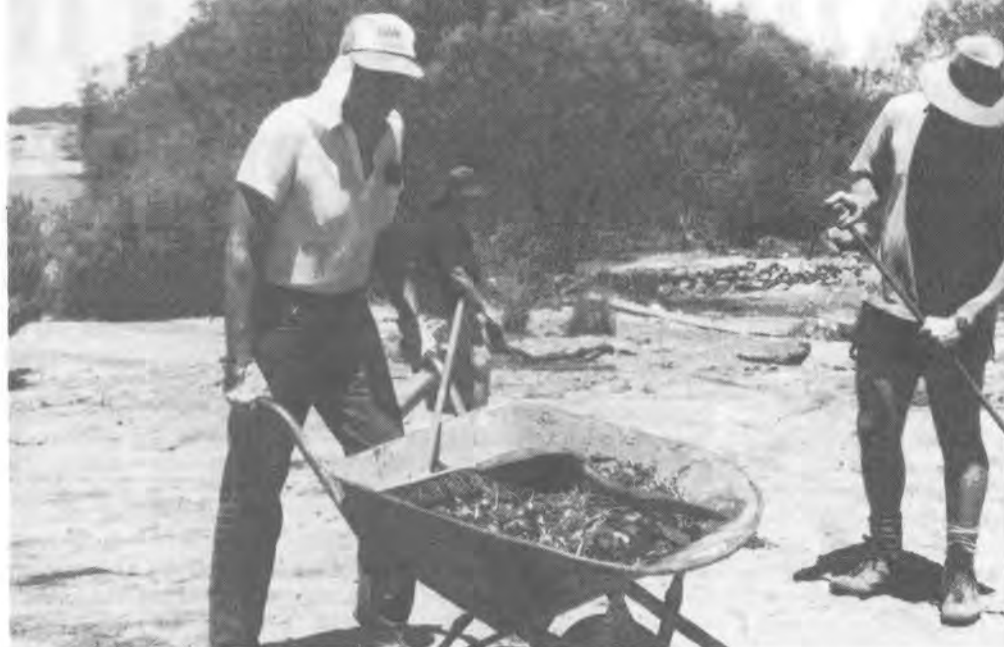
Broken glass by the barrow load! Richard Eaton from Boulder Lions Club pushes while Ben Carr from Australian Conservation Volunteers rakes.
