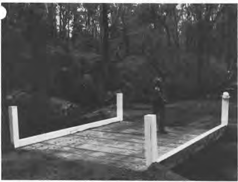
Pictured here are photographs taken of one such bridge by Jarrahdale district staff.
