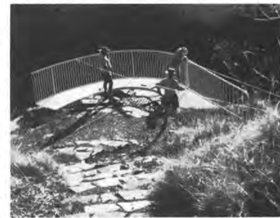
Sections of the safety railing being fitted on-site at Joffre Gorge in the Karijini National Park.
