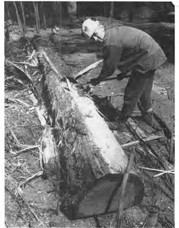
Collie forest workman Dean Guest removes bark from a log that will become part of a bridge at Honeymoon Pool.
