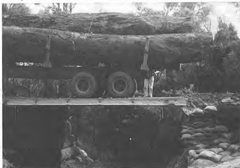
The new bridge deck undergoes weight-bearing exercises. Photo by Des Donnelly
