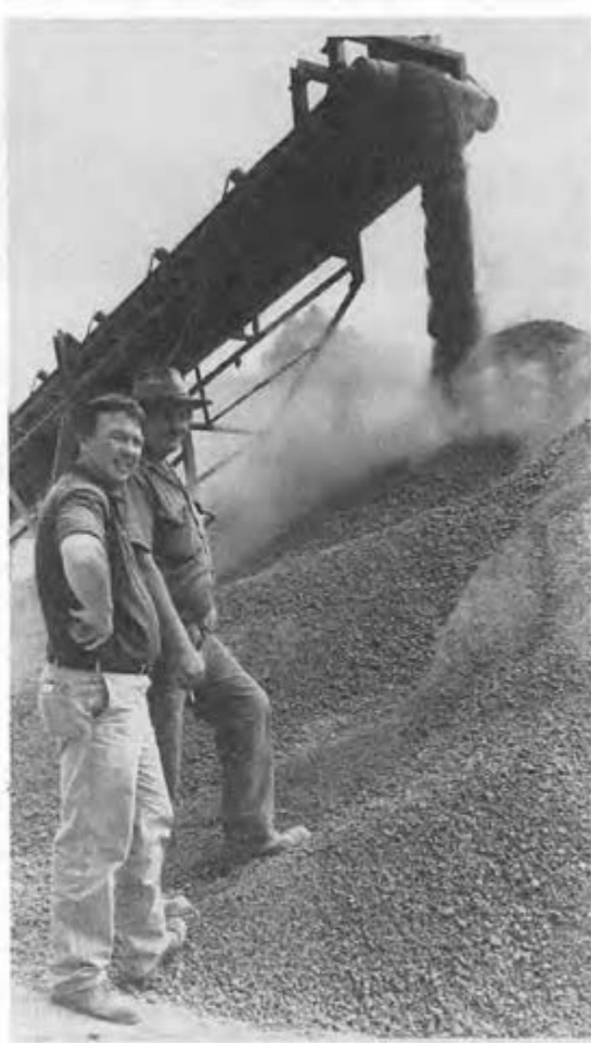
CALM Margaret River district officer Brad Commins and Quarry Park site manager George Bem inspect outcome of the new quarrying method. Photo by Gabrielle Adams, courtesy Busselton-Margaret Times
