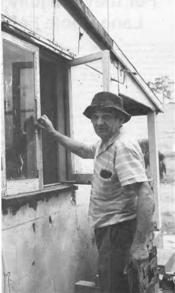
Technical advisor Helmut Hiddel checking glazing work at the homestead. Photo by Carolyn Thomson
